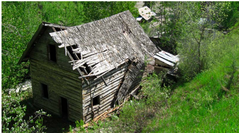
Old Vance house next to Telegraph Creek
