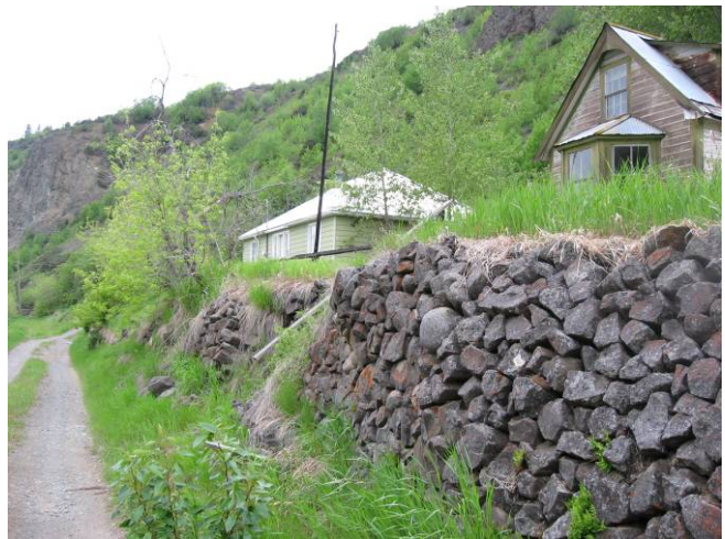
Basalt rock retaining walls.
