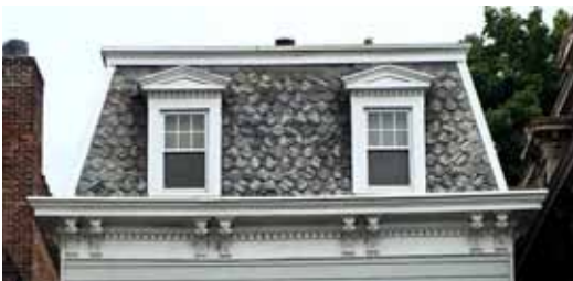
Distinctive Mansard Roof: Dual-Pitched, and Hipped, with slate roof and dormers.
