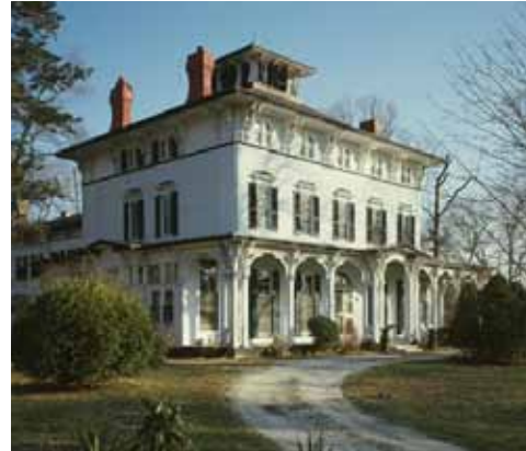
George Allen House Cape May, NJ HABS
