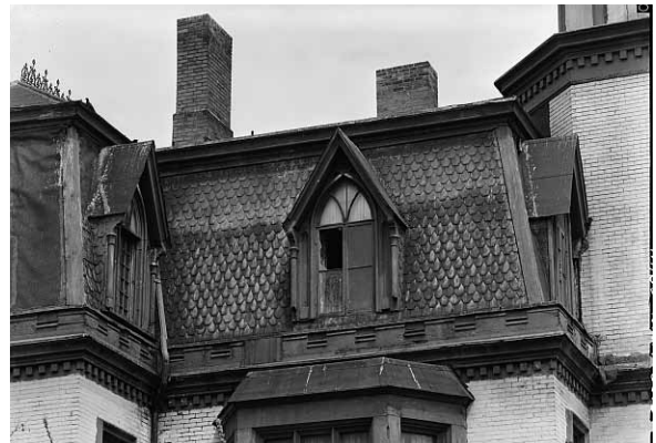
Cary House - Buffalo, NY - HABS Another fine example of a Mansard roof.
