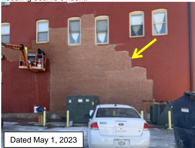
Photograph indicates area of repaired (unpainted) brick from outside building.
