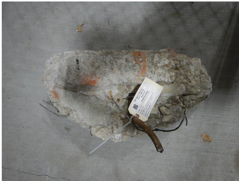
Appendix D – Photograph 4: Exemplar concrete floor slab material.
