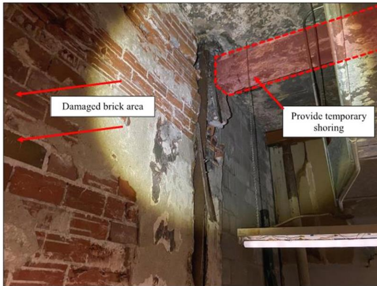
Photo 2 – Second Beam to Support
